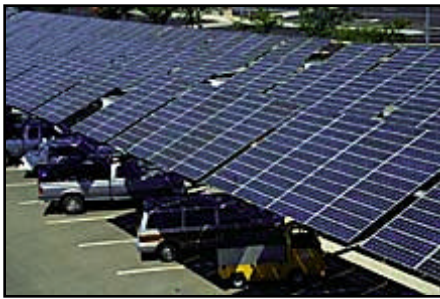
Above: Solar ports over parking lots: protect cars and parking surface and generate electricity
