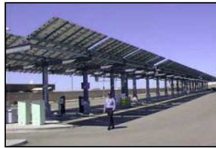
Above: Solar ports over parking lots: protect cars and parking surface and generate electricity
