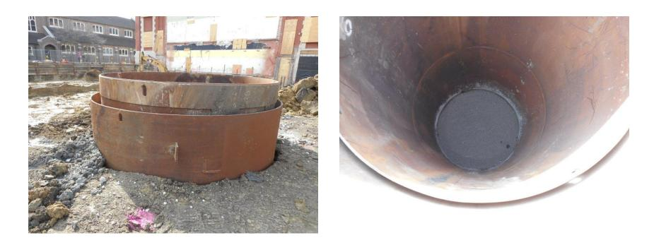
Deep sump pit drilled/sleeved in order not to impact deep foundation installation, the casing is 12' diameter and 20' deep.
